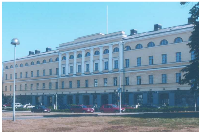
Photograph 1. Ministry of Foreign Affairs of Finland, old sailor barracks, north elevation (sea side). Basement and three stories.
