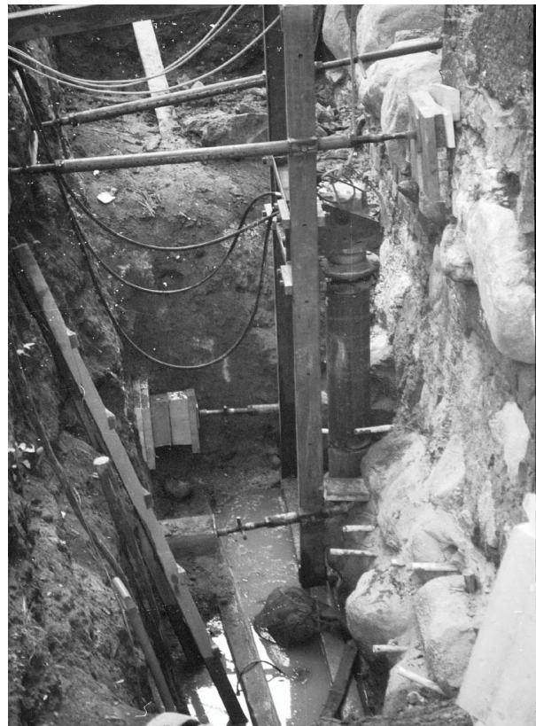
Photograph 1. Simple screw equipment for spiral drilled piles.
