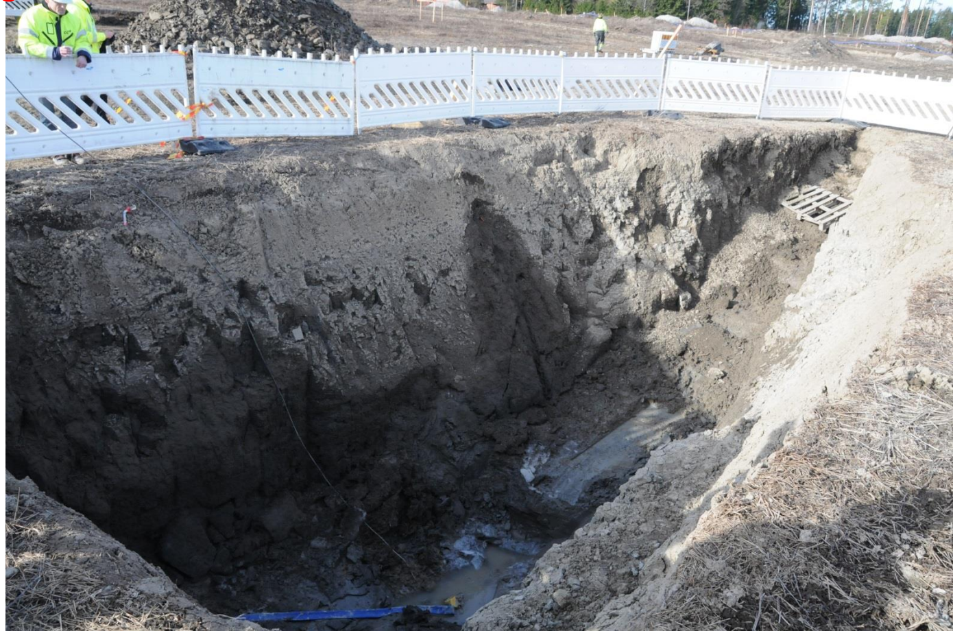
Figure 10. Unbraced test trench. Underlying soft clay is flowed towards the trench
